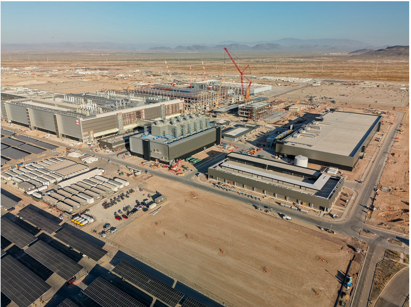
Image: TSMC Fab 21 under construction in Phoenix, Arizona (November 2023).
