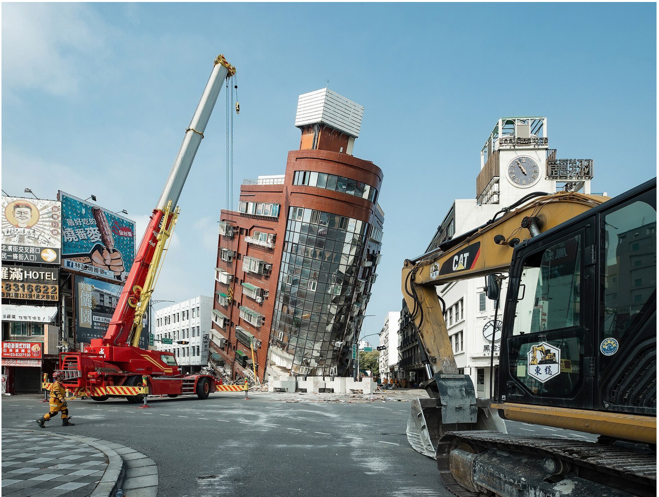
Image: Rescue workers and equipment near the dangerously-leaning Uranus Building on Xuanyuan Road in Hualien City, in the immediate aftermath of the April 3, 2024 Hualien earthquake. (Image source: ROC Presidential Office / Wikimedia Commons )
